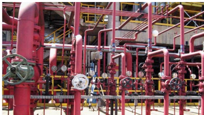
3D Laser Scanning in chemical facility
